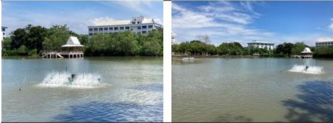
Aerated Lagoon and Paddle Wheel Aerator in NPRU
