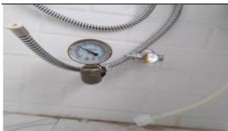
Surveying and testing the water pipe system in the building
