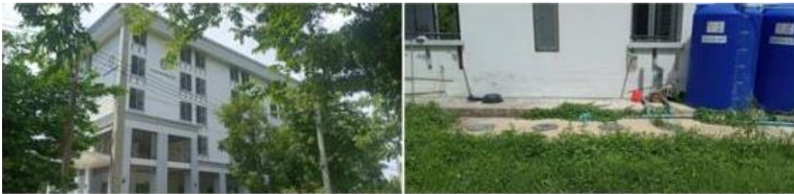
Building and service capacity of the building's septic tank
