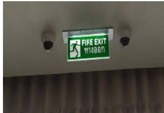
[S3] CCTV system.
